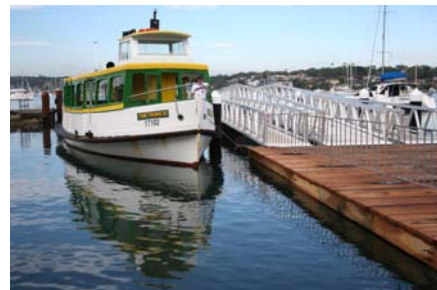
The new wharf in Gunnamatta Bay nearing completion.
